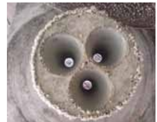
Inside the unit is clean and fully operational.
